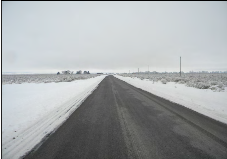
LOOKING NORTHERLY AT 18150 WEST
