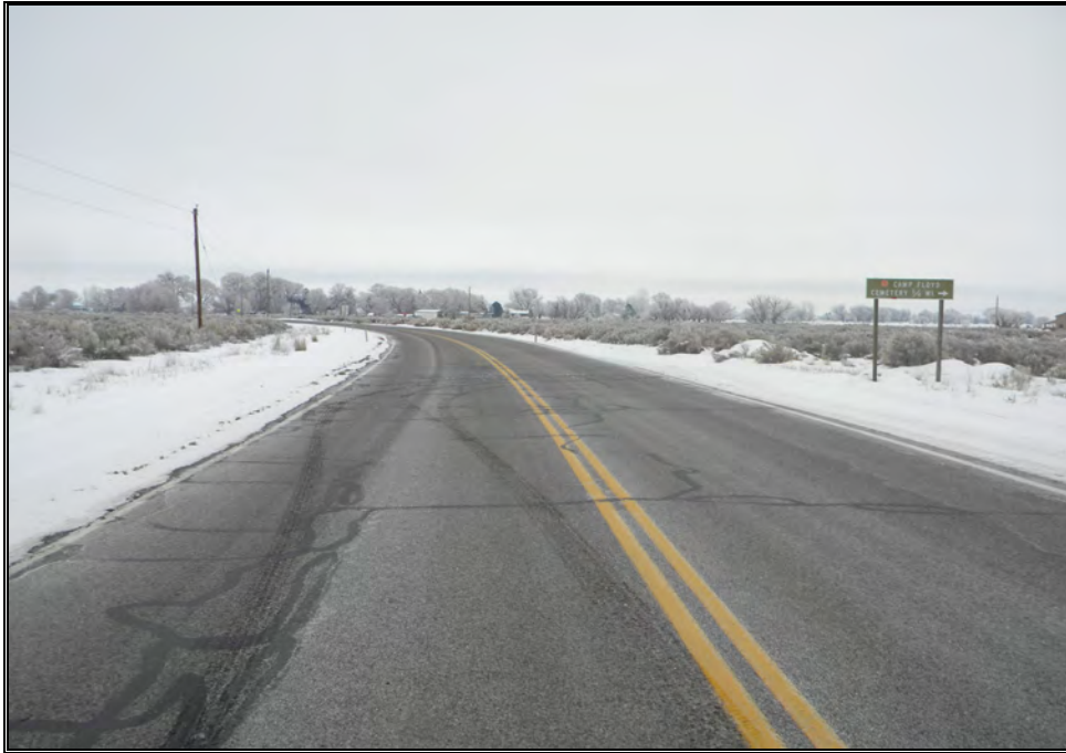
LOOKING EASTERLY AT HIGHWAY 73
