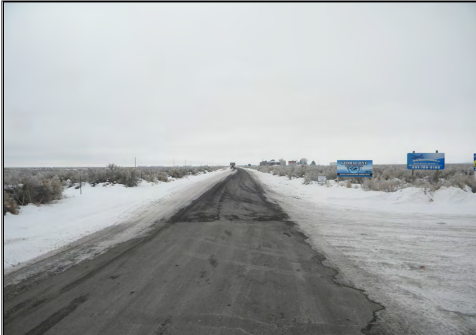
LOOKING SOUTHERLY AT 18150 WEST
